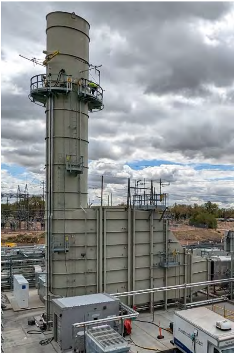
SCR ready exhaust (pre-installed ammonia nozzles)
