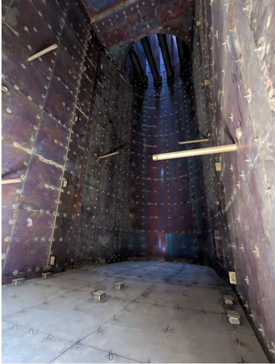
SCR ready exhaust (pre-installed ammonia nozzles)
