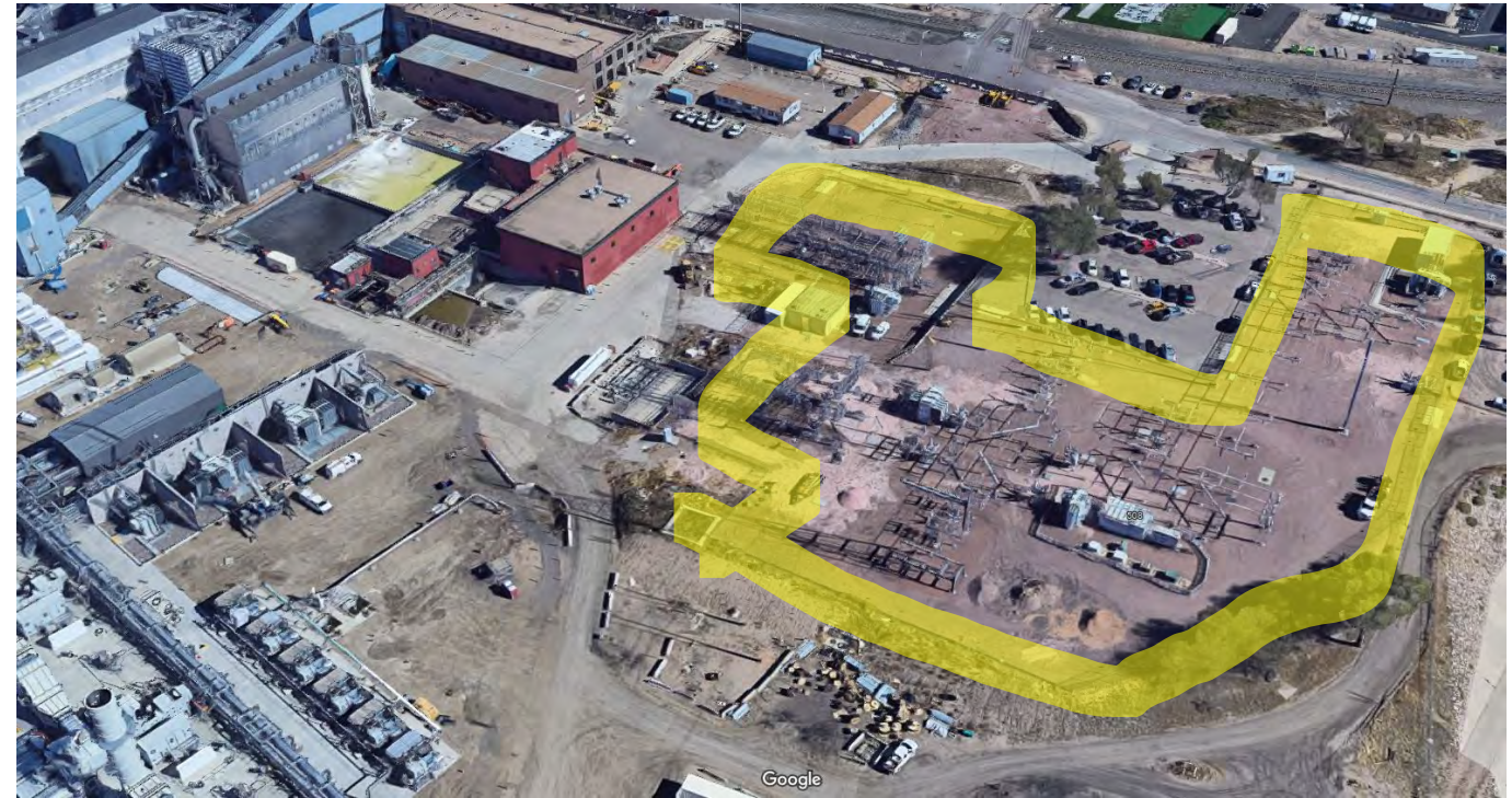
South Plant Substation
