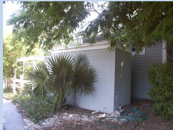
Florida House Cistern
