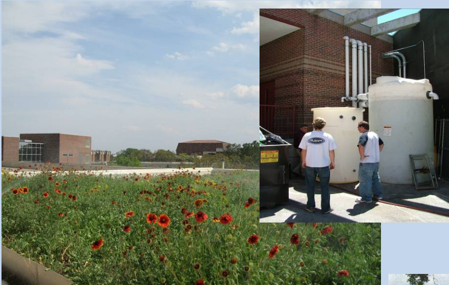
UCF Green Roof/Cistern
