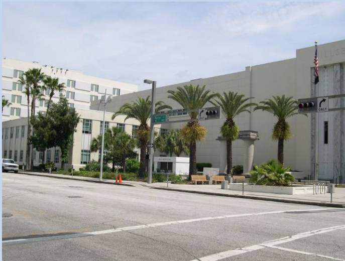
Cistern at the Hillsborough County Courthouse
