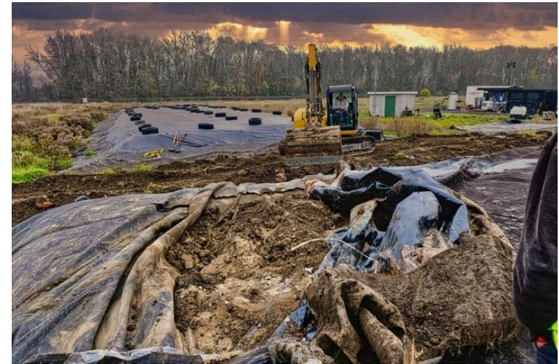
Through laboratory and field studies, smoldering-based thermal treatment was demonstrated to destroy per- and polyfluoroalkyl substances, the “forever chemicals” in soils. Of utmost importance to the DoD funding agency, ESTCP and SERDP, was understanding the mass balance of PFAS destruction.
