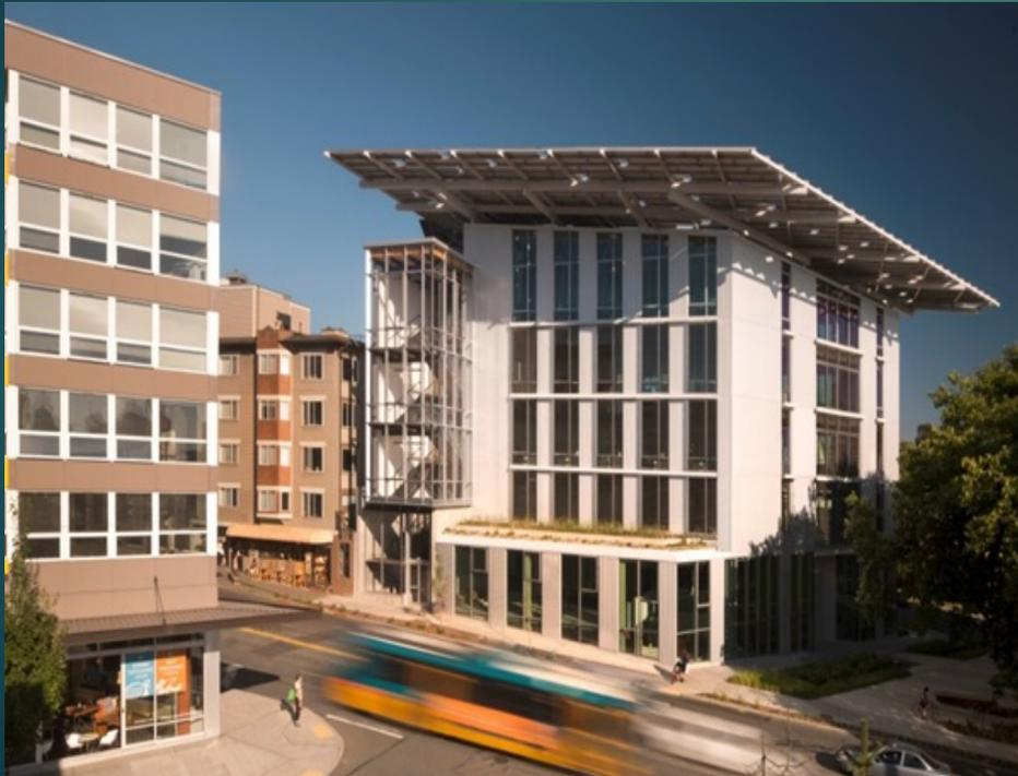
The practices incorporated in the building include energy conservation and geothermal energy, roof solar panels, rainwater harvesting, waterless toilets, black water and solids aerobically composted, gray water treated by wetland and reused. (Pictures credit Nick Lehoux) .
