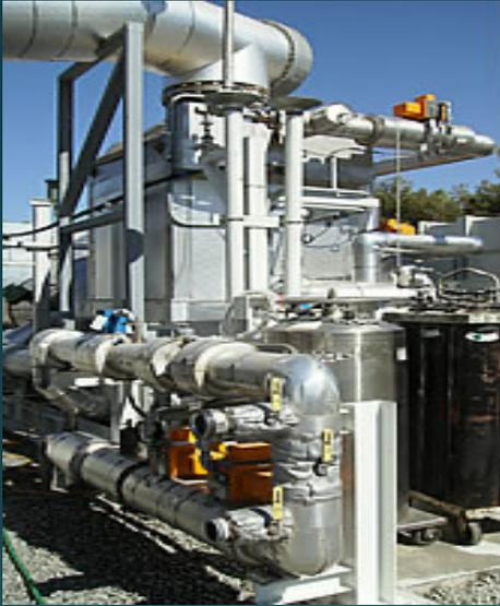
1.2 MW DFC 1500 Fuel cell MCFC power plant with internal biogas reforming manufactured by FuelCell Energy installed in Riverside, CA water reclamation plant.
