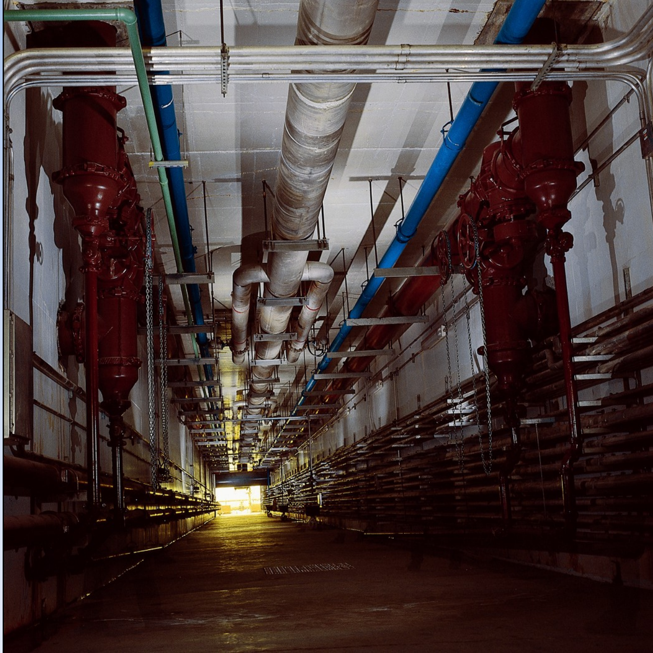
Pipe Gallery Tunnel with Internal Recycle & Air Piping
