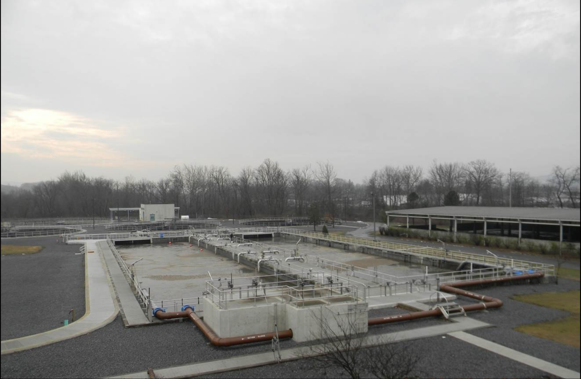
Existing Aeration Tanks Converted to NRT Reactors and Adjacent Step-Feed Channel to Last Oxidic Zone
