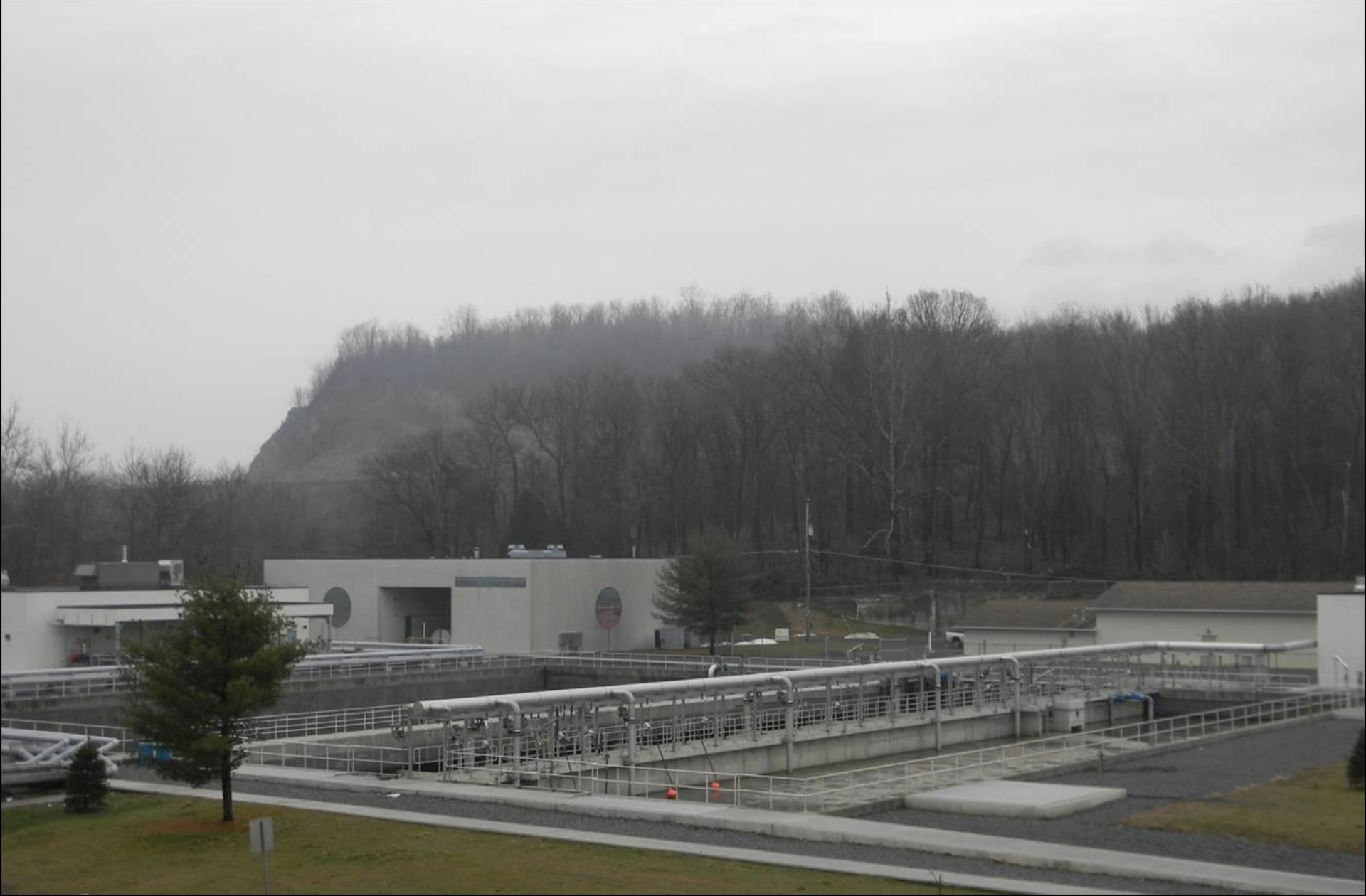
Conversion of South Equalization Tank to NRT Reactors
