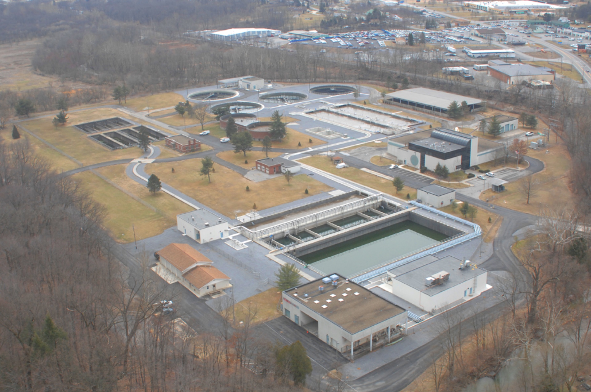
Upgraded Westerly WWTF
