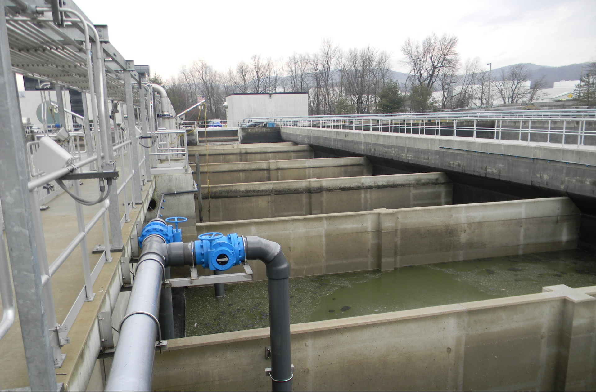
Retrofitting of Existing Equalization Tank to NRT Reactor
