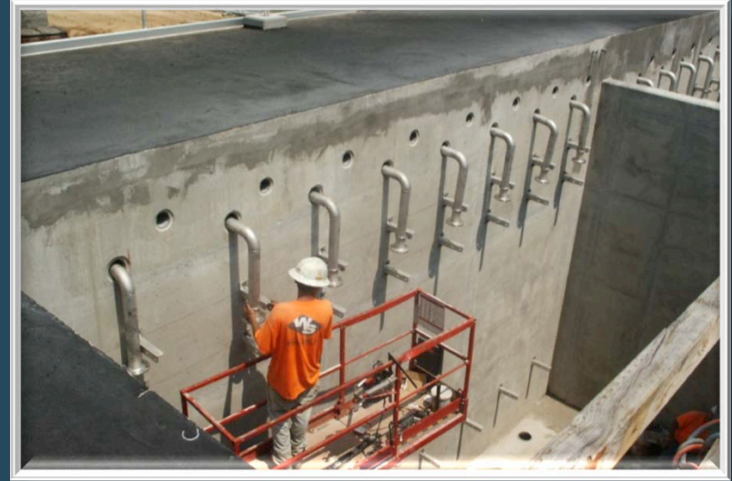
MBT Tank During Construction
