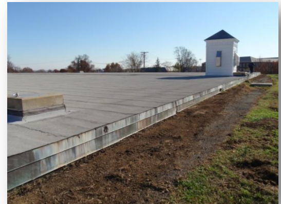
West End of Reservoir from Northwest Corner
