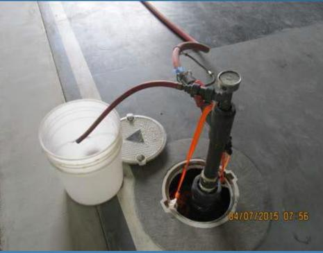
Concrete was removed to install conveyance piping and an SVE well.
