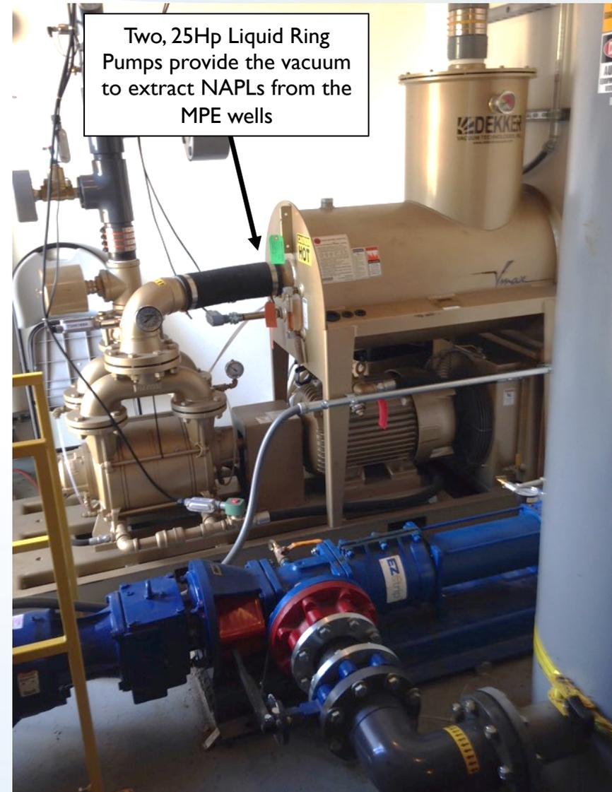
Two, 25Hp Liquid Ring Pumps provide the vacuum to extract NAPLs from the MPE wells
