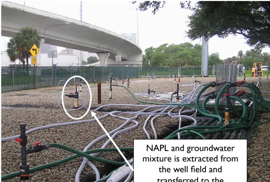
NAPL and groundwater mixture is extracted from the well field and transferred to the treatment components
