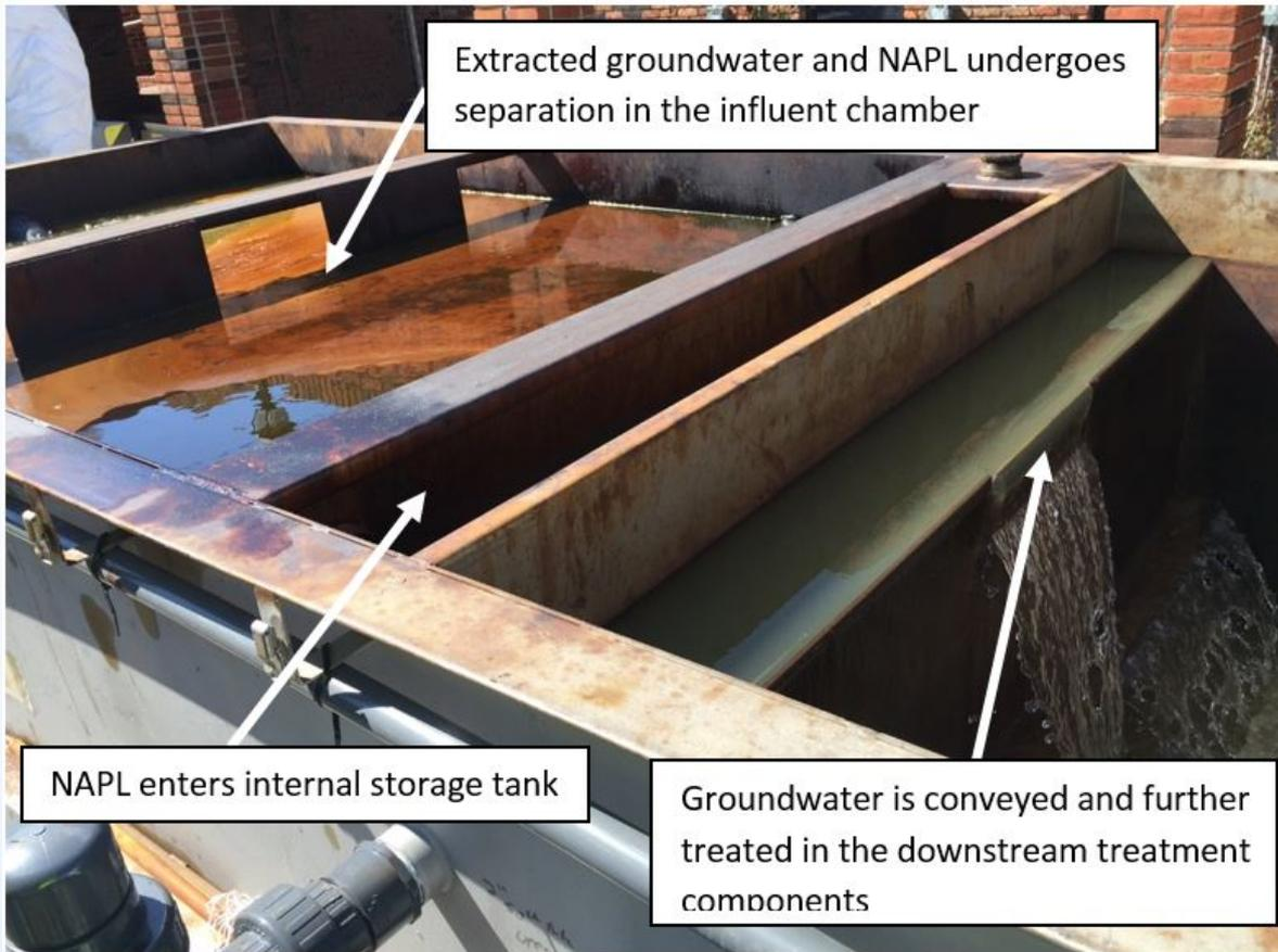
Extracted groundwater and NAPL undergoes separation in the influent chamber
