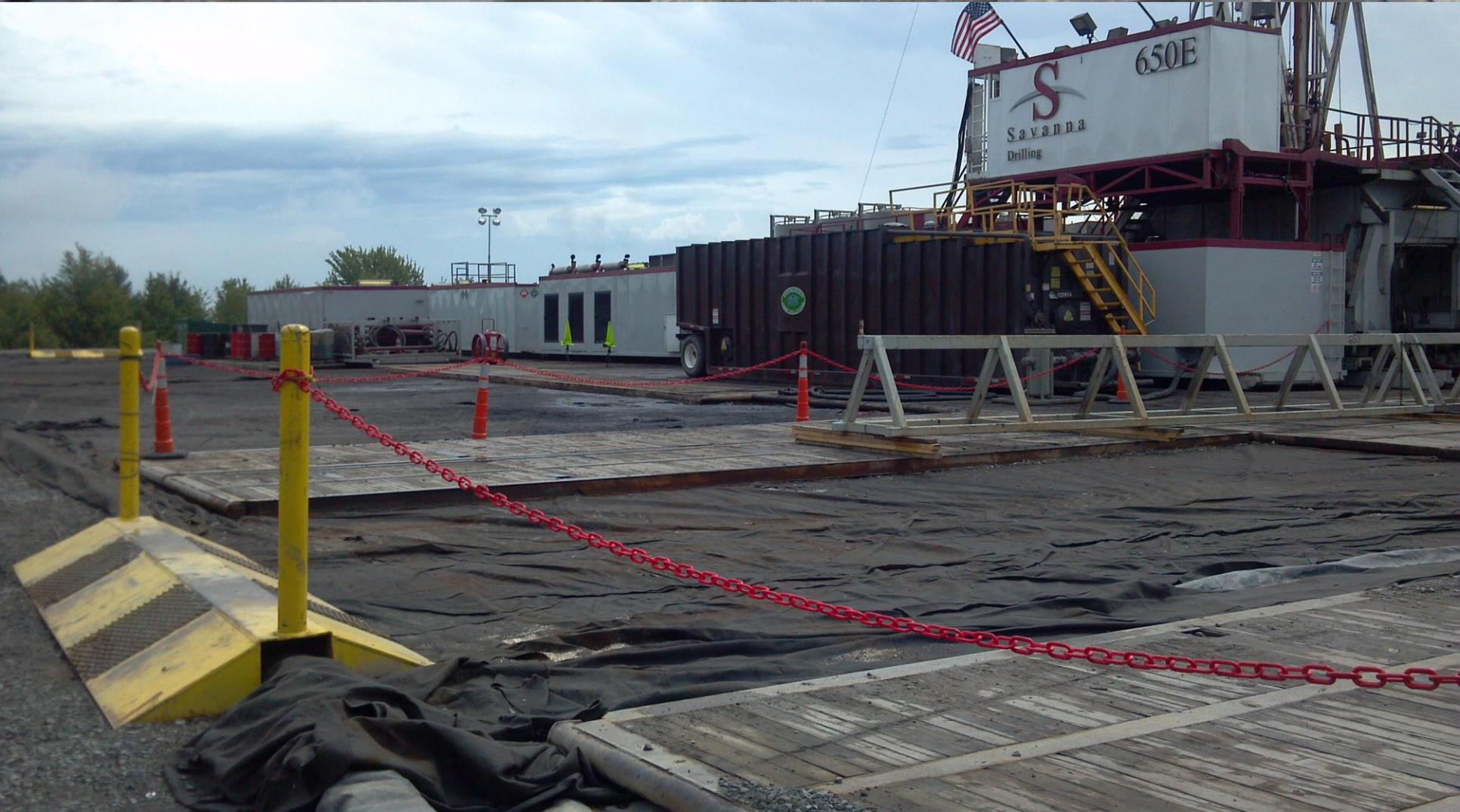
Potential for soil or groundwater contamination is minimized with lined well pads.
