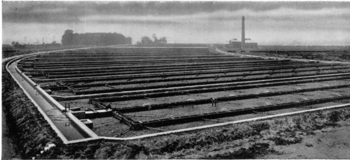
LEICESTER SEWAGE PURIFICATION WORKS, 12 ACRES IN EXTENT—E. G. MAWBAY, Esq., M.I.C.E., CITY ENGINEER
