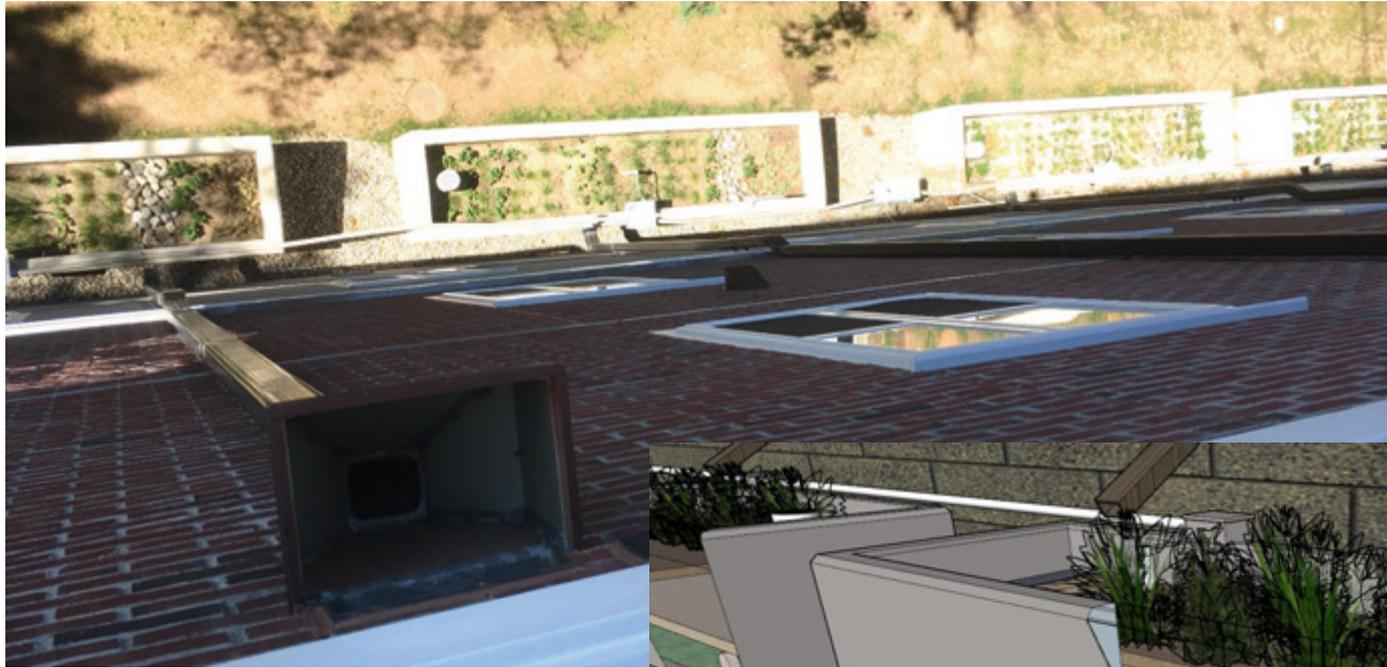
Planter acts as a **bioretention cell** to manage roof runoff
