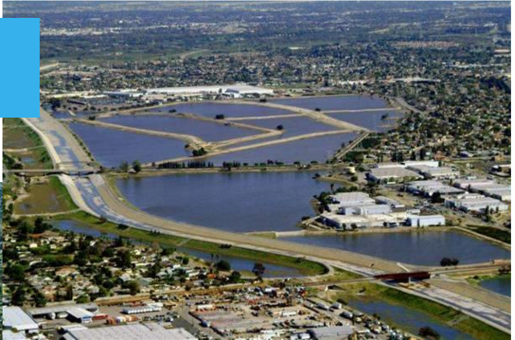
Rio Hondo spreading basins
