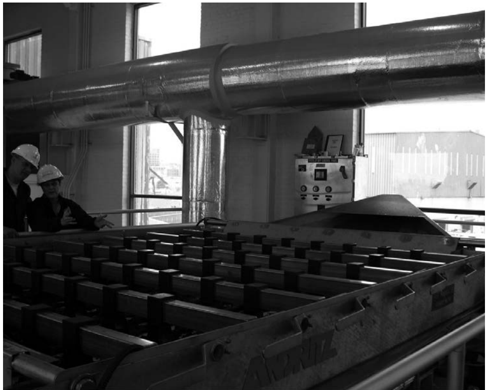
FIGURE 6 BELT FILTER PRESSES
