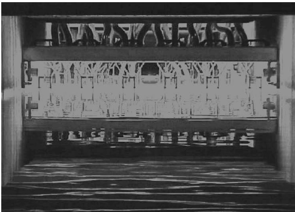
FIGURE 4 ULTRAVIOLET DISINFECTION
