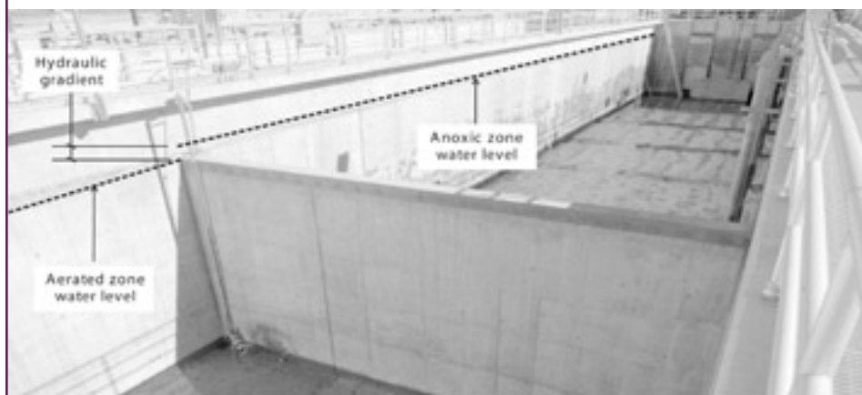
FIGURE 8 Requirements for Correct Baffle Design and Construction
