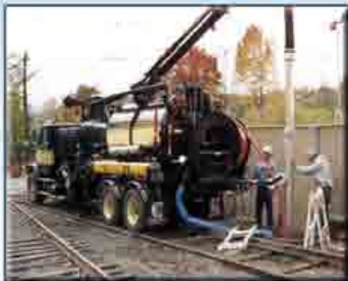
SEWER CLEANING: High-Pressure Jetting / Power Bucketing: Single and double-pump, jet-vac combination units with line jetting capabilities of 175 gpm / 2,500 psi literally scour sewers clean. Specifically sized buckets quickly and thoroughly remove all debris from severely clogged sewer lines.
