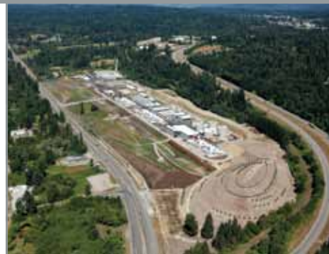
Brightwater has redefined the municipal wastewater treatment plant and is setting standards of practice for wastewater treatment and reclamation around the country.
