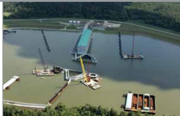
The WCC Pump Station is a truly unique structure. It is longer than two football fields, and over 100 feet high. When the sector gate is closed in advance of an impending storm, the pump station will prevent substantial flooding in the West Bank area by discharging upstream drainage to the flood side of the barrier.
