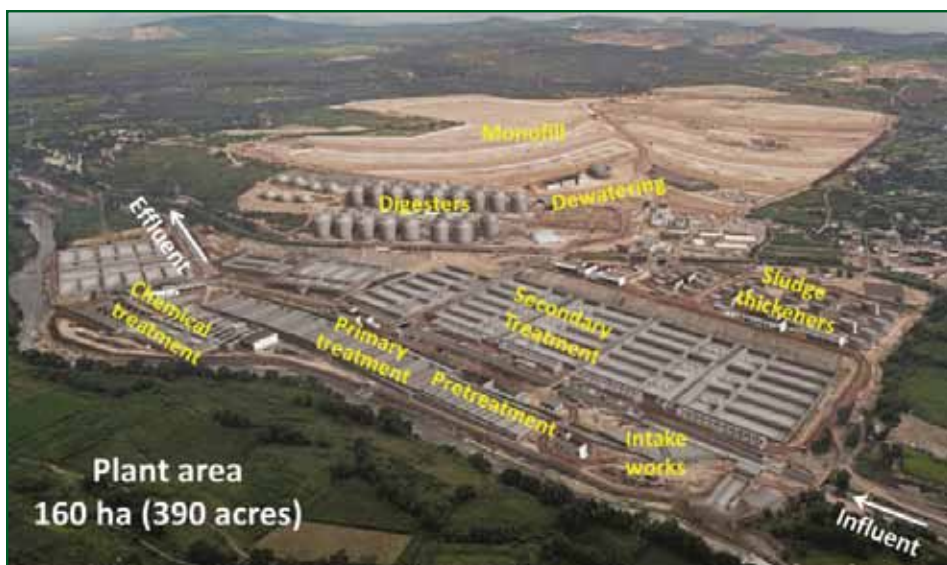
Figure 5: Atotonilco WWTP, under construction Photo credit: Aguas tratadas del Valle de México, S.A.
