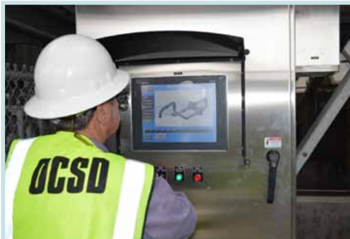
PLC display for the emissions control system showing system configuration.
