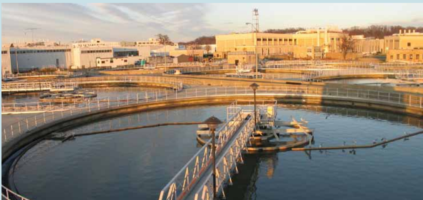
BOTTOM Primary treatment to redirect carbon to anaerobic digestion.
