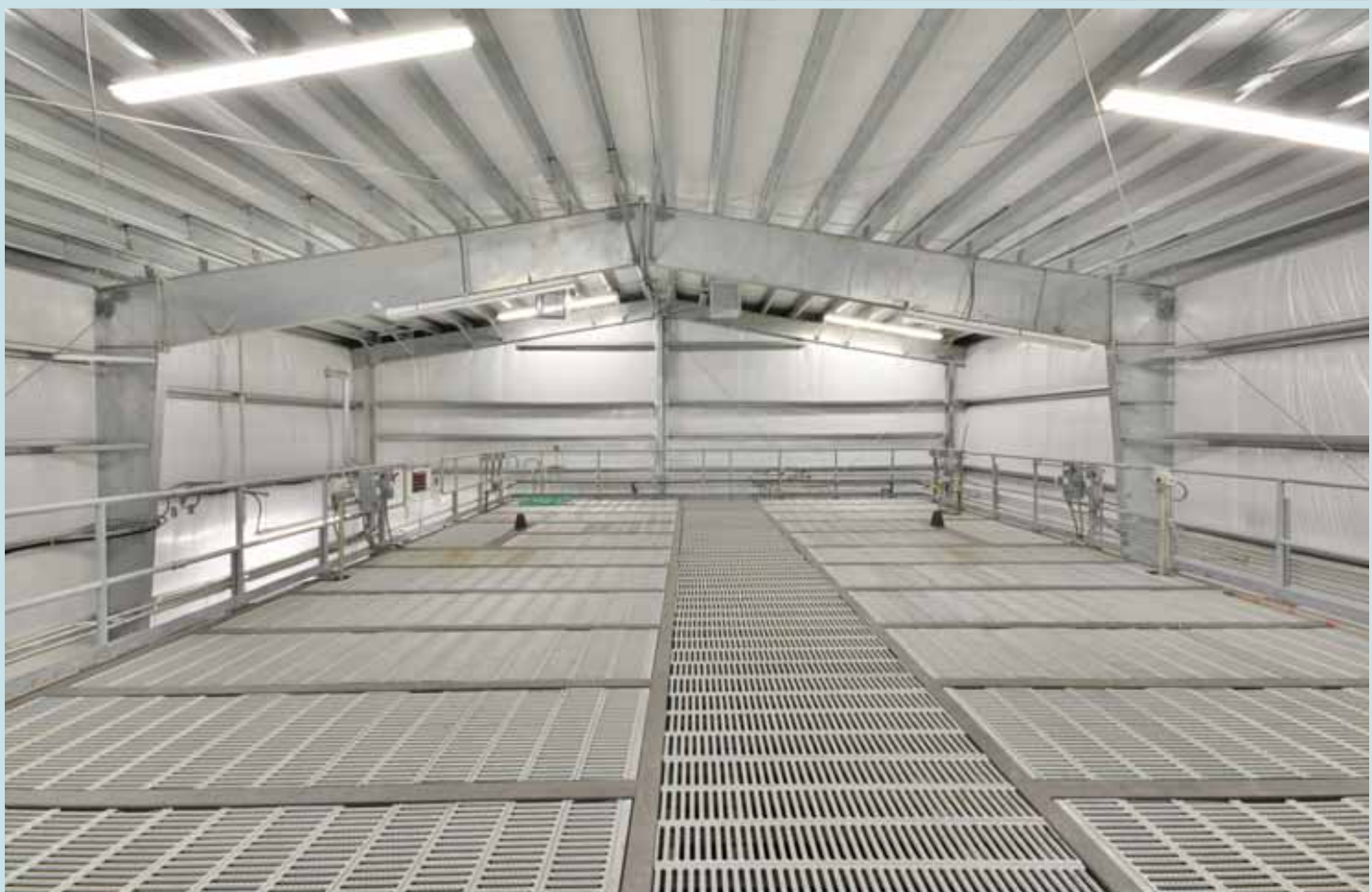
BOTTOM Wastewater treatment plant interior - Treatment units below grating
