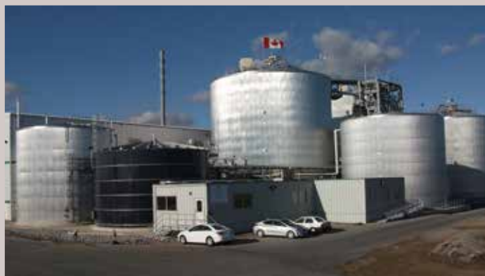
The City of Toronto owns two organics processing facilities that digest collected organic material through anaerobic digestion.
