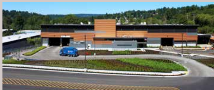
Solid waste handling buildings are considered essential public facilities in Washington State. Since Factoria Recycling and Transfer Station provides a critical function in the community, especially during recovery from natural disasters, the building was designed for immediate occupancy following a natural disaster, including a major seismic event.
