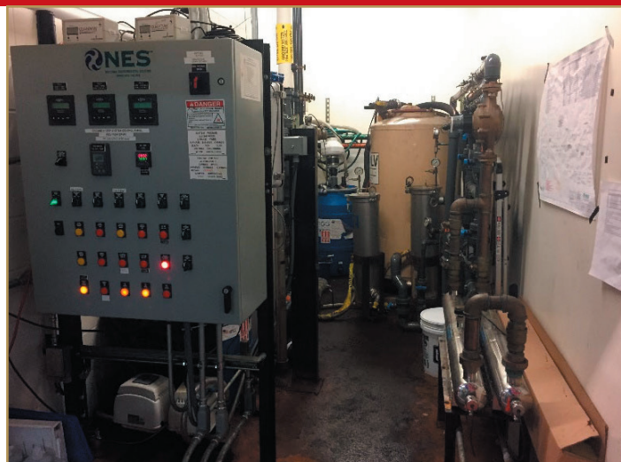
7 Years Later. The groundwater treatment system operated continuously for the above 7 years. Modifications were made over the years as adjustments to treatment were needed.
