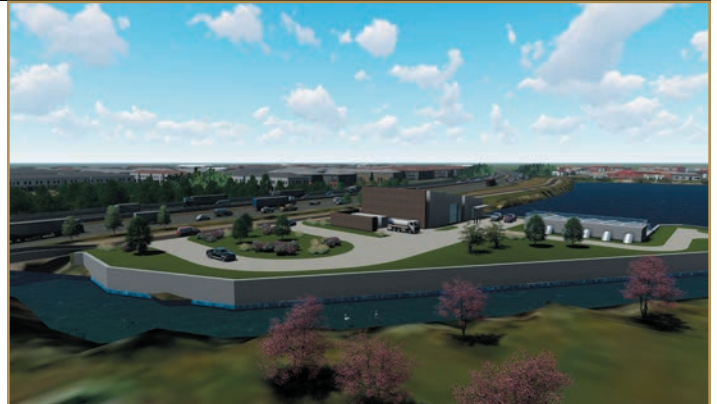
The Windsor Woods stormwater pump station located on Thalia Creek will lower upstream water levels prior to storm events and provide up to 750 cubic feet per second (cfs) of capacity to maintain water levels to meet the established level of service.
